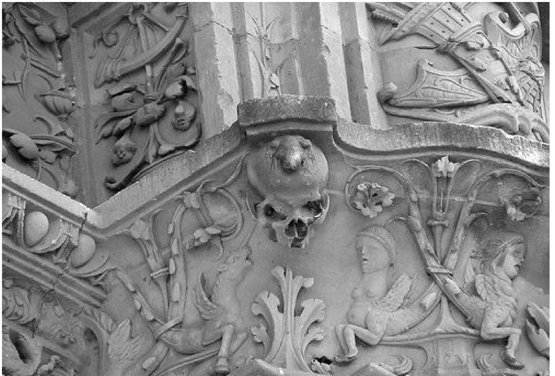
DETAIL ON THE UNIVERSITY FAÇADE / DETALLE
