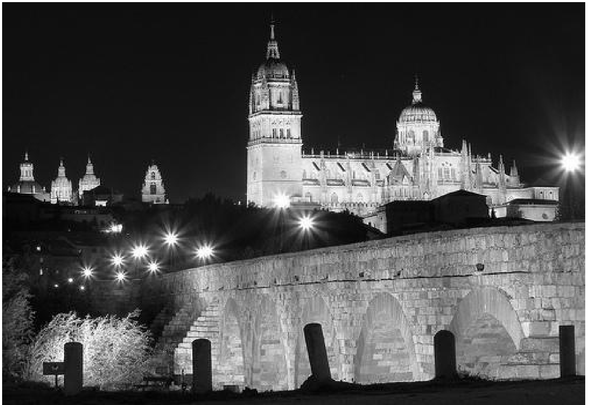
ROMAN BRIDGE 1st Century / PUENTE ROMANO
